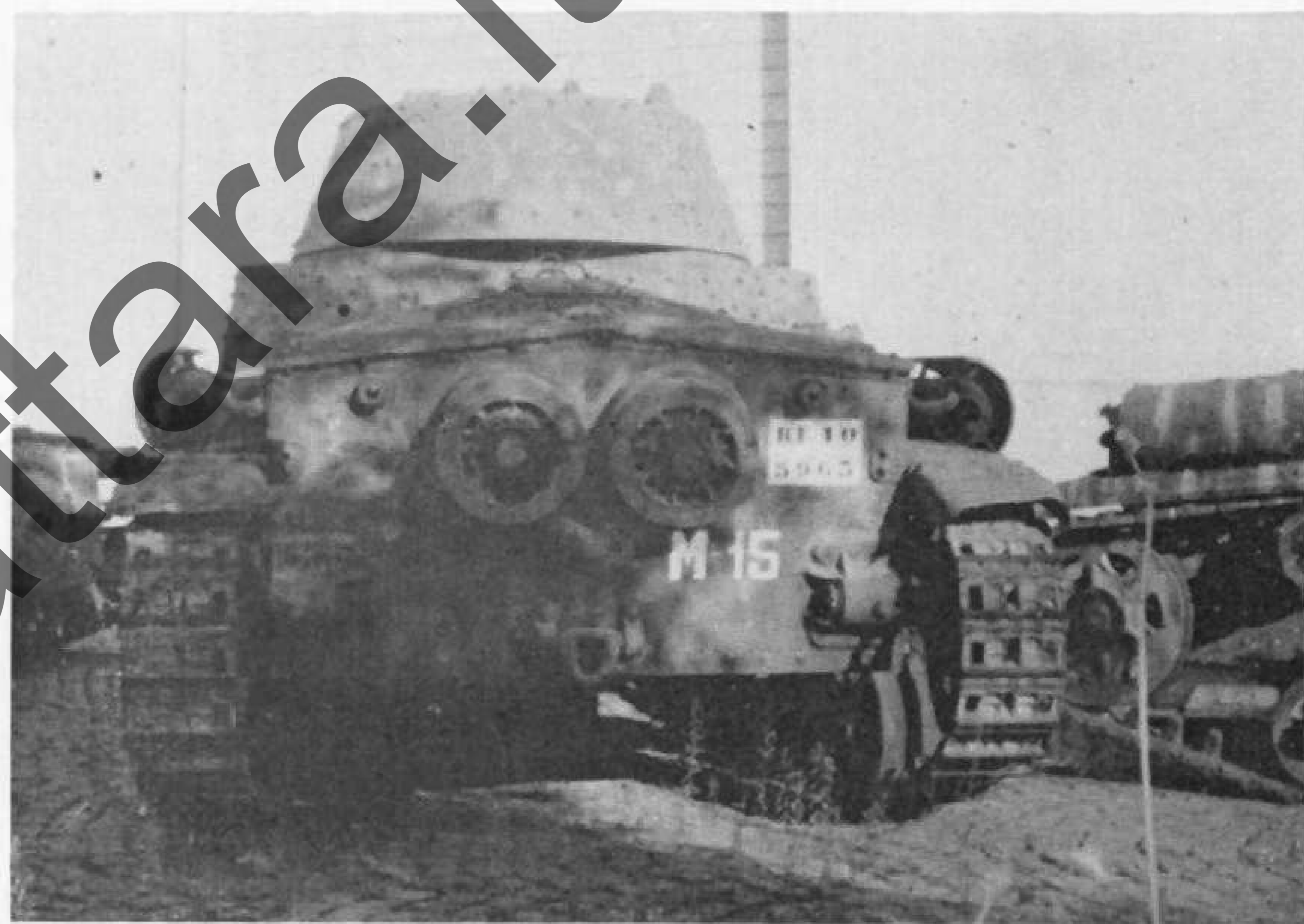
Three views of M 15/42. Note the larger gun, access hatch moved to right side and modified rear hull.
